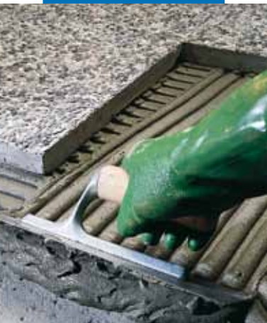
External installation of relief terrazzo "graniglie" tiles
