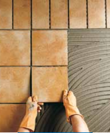
External installation of klinker tiles
