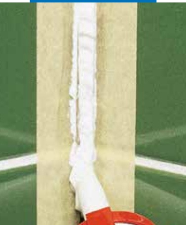
Application of Mapesil AC
