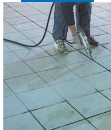
Sealing ceramic tile floor with Mapesil AC
